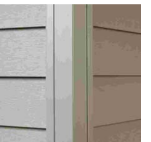
Traditional corner post with foam insert.
